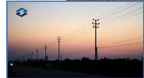
132 KV (29m high)
